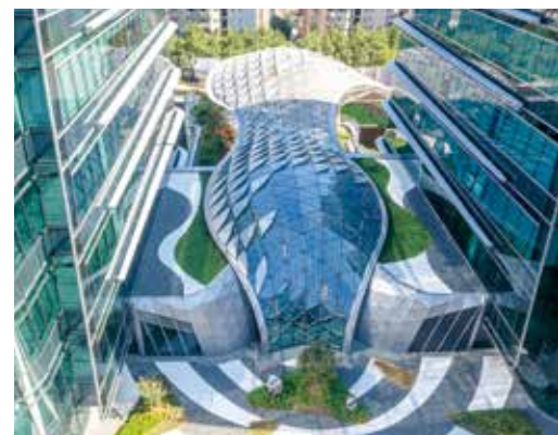
One ITC includes two office towers and a shopping mall 國貿匯由兩幢寫字樓和一個商場組成
