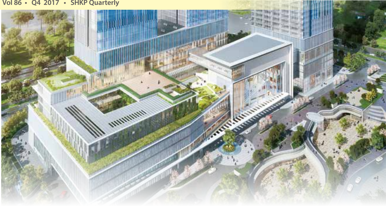
Located in Hexi Central Business District, Nanjing IFC will be atop Metro Yuantong Station 南京國金中心座落於河西中央商務區，為地鐵元通站上蓋物業
