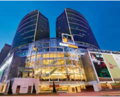
Excellence in Facility Management Grand Award for office buildings and silver Theme Award – Energy Management to Grand Central Plaza 新城市中央廣場在「卓越設施管理獎」中，榮獲卓越大獎（商業樓宇）及能源管理主題獎銀獎
