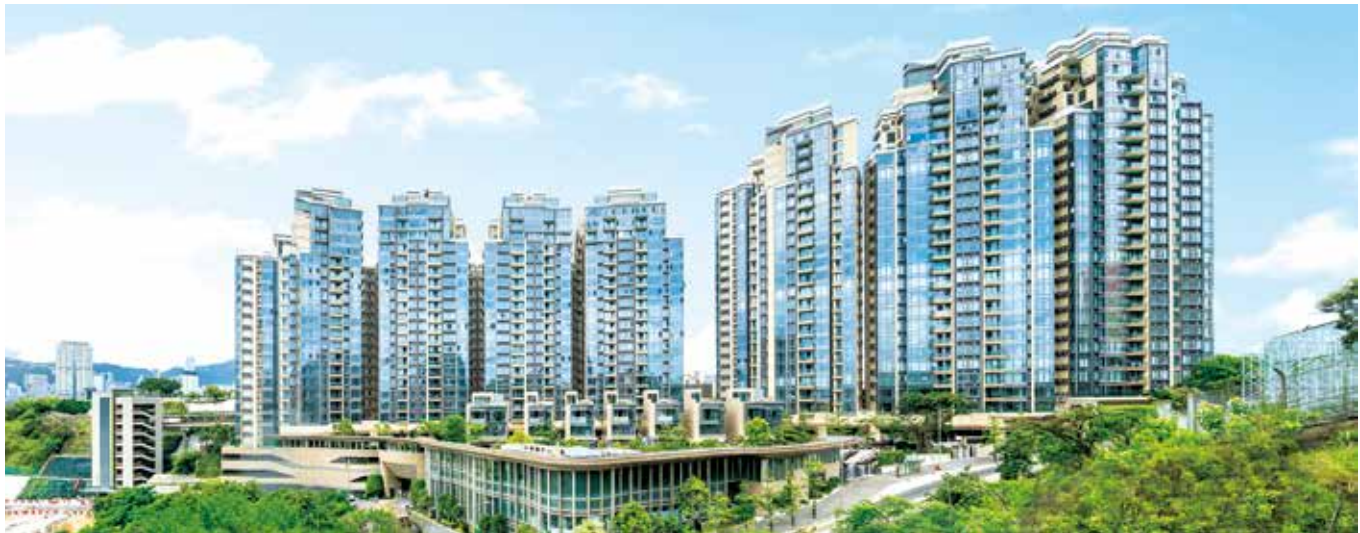
This photograph was taken at the Development on 29 June 2016. It has been processed with computerized imaging techniques and is for reference only. 以上圖片於2016年6月29日於發展項目現場實景拍攝，並經電腦修飾處理，僅供參考。
