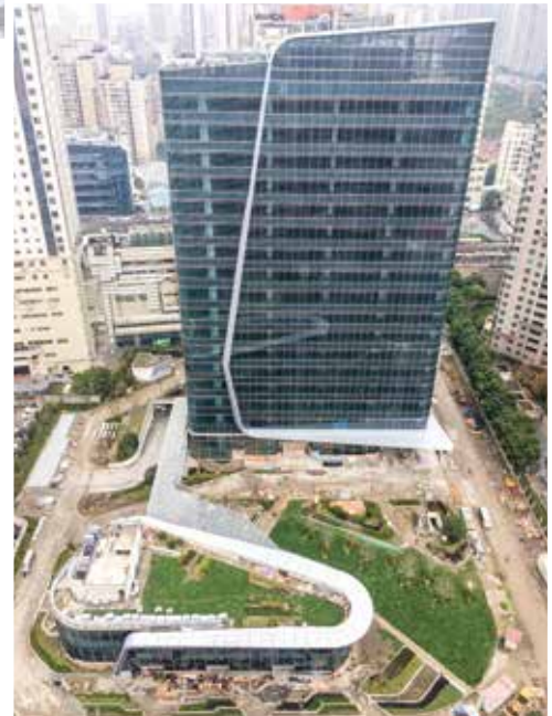
Phase 2 of ITC will complete by this second half 徐家汇国贸中心二期快将于今年下半年落成
