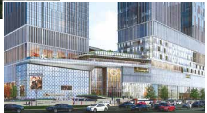
The Nanjing IFC mall will feature international top-tier tenants and new comers to Nanjing
