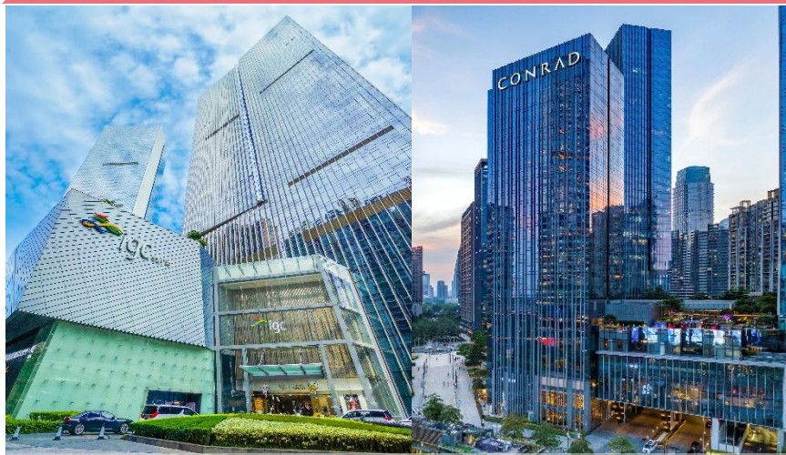
IGC mall & Conrad Guangzhou hotel at Tianhui Plaza, Zhujiang New Town CBD, Guangzhou
