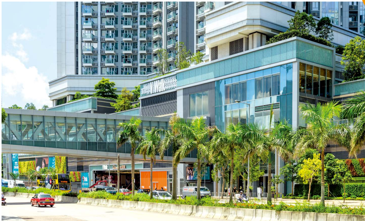
V Walk, above MTR Nam Cheong Station, will have all-day indoor walkways and bridges conveniently connecting it to nearby major residential developments V Walk位處港鐵南昌站上蓋，並設有全日開放的室內行人通道及天橋連接附近大型住宅項目，出入方便
