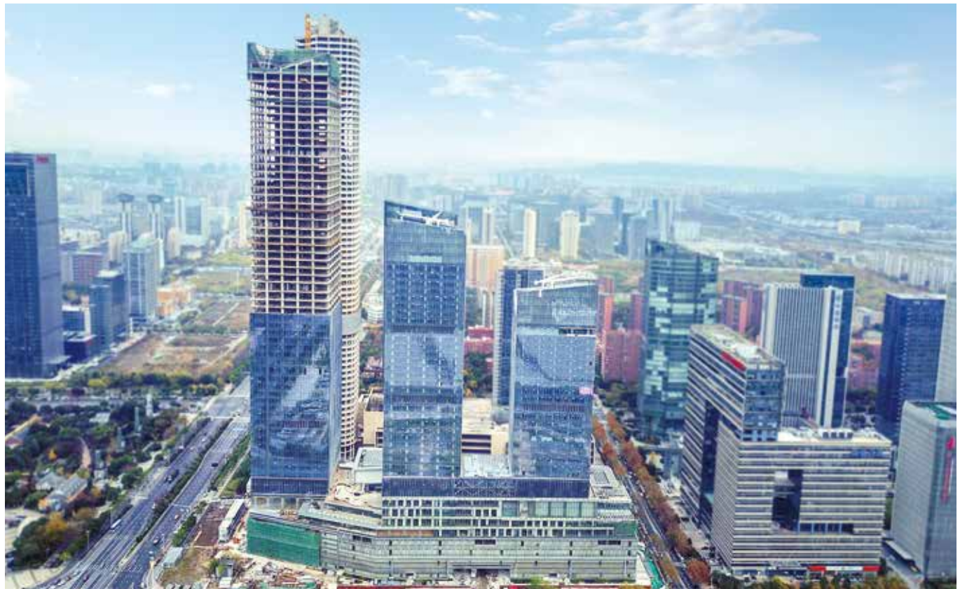
Nanjing One IFC is currently carrying out pre-handover, final inspections (centred). The shopping mall is currently carrying out interior work (podium). The hotel (right) and Nanjing Two IFC (left) have been topped out (site photo taken on 5 December 2018)
