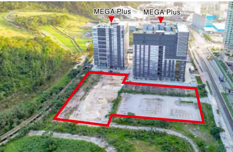
SUNeVision's new data centre site in Tseung Kwan O sits next to the flagship facility MEGA Plus 新意网新增位于将军澳的数据中心地皮，毗邻为旗舰数据中心MEGA Plus
