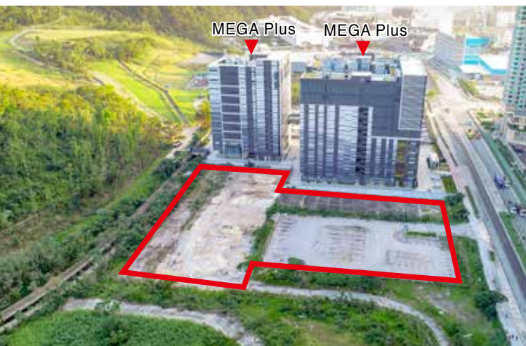
SUNeVision's new data centre site in Tseung Kwan O sits next to the flagship facility MEGA Plus 新意網新增位於將軍澳的數據中心地皮，毗鄰為旗艦數據中心MEGA Plus
