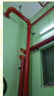
更換消防上水喉 Replace existing F.S. hydrant pipe
