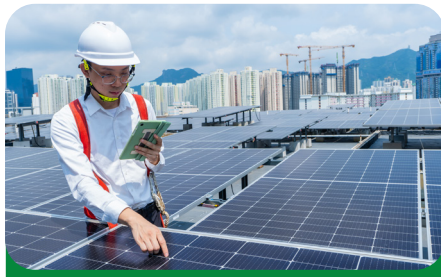
Solar systems at Tonic Industrial Centre
