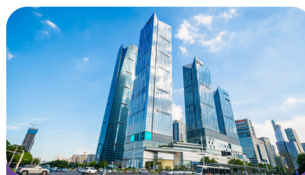
Nanjing IFC, located above Nanjing Metro Yuanlong Station, connects seamlessly to two existing metro lines
