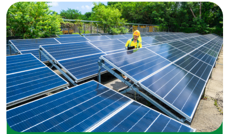
Solar farm at Sai Sha construction site
