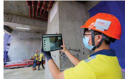
• A worker wears a Smart Helmet integrated with IoT sensors and GPS tracking
