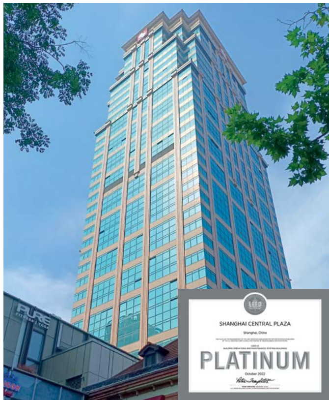
Shanghai Central Plaza, the Group's third landmark development in Shanghai, received LEED v4 O+M:EB Platinum certification 上海中環廣場榮登集團旗下第三個獲得 LEED 既有建築鉑金級認證 (LEED v4 O+M:EB Platinum) 的上海地標項目
