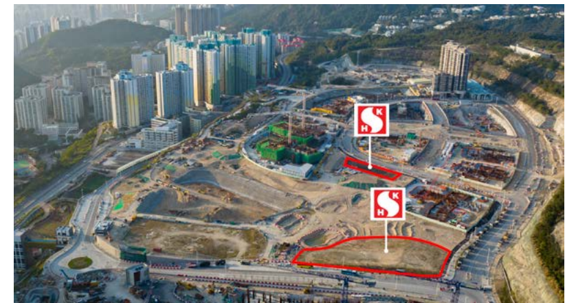
The Group plans to develop community shopping centres on the commercial sites near Anderson Road 集團計劃在安達臣道附近的商業用地興建社區購物商場
