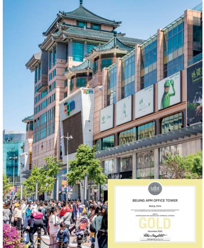
The Beijing APM Office Tower received LEED v4 ID+C:Commercial Interiors Gold certification 北京APM 写字楼荣获LEED商业室内金级认证 (LEED v4 ID+C:Commercial Interiors Gold)
