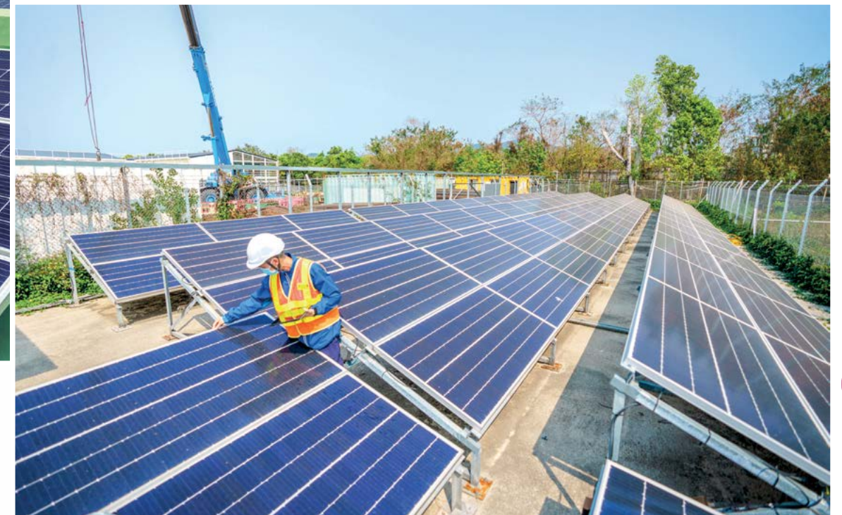
The large-scale residential project in Shap Sz Heung, now under construction, has Hong Kong's first solar energy system built on a temporary site, with 114 solar panels installed 正在兴建中的十四乡大型住宅项目，设有全港首个在临时工地搭建的太阳能发电系统，该处共安装了114块太阳能板
