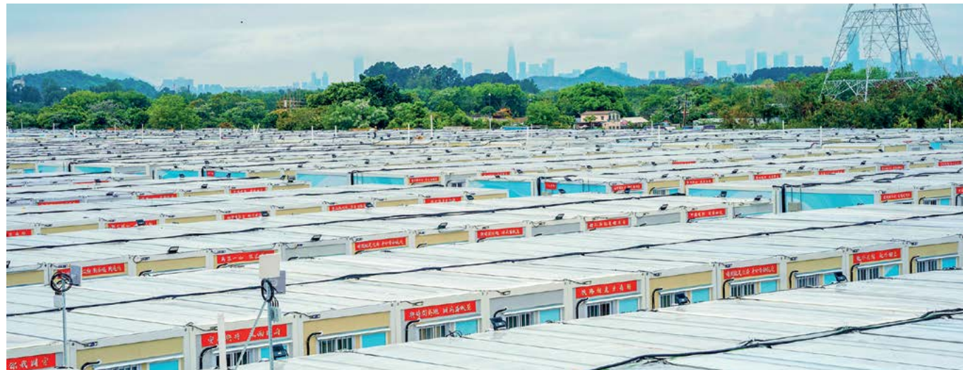
Community isolation facility in Tam Mi, Yuen Long was completed and handed over to the government for use 元朗潭尾社區隔離設施已落成，並正式交付予政府營運
