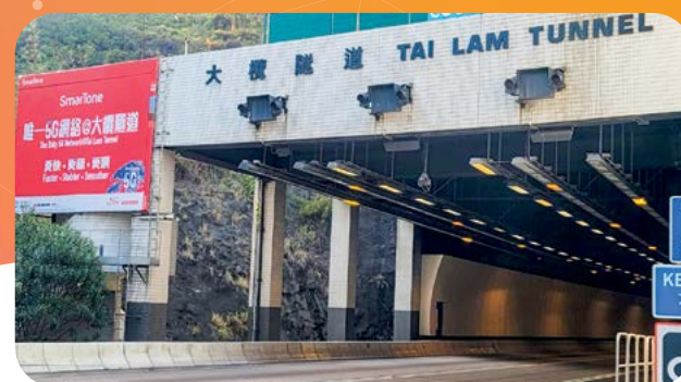
The Tai Lam Tunnel utilises the 5G SmarTransport Safety Monitoring System, which enhances traffic safety and operational efficiency 大欖隧道採用5G智慧交通安全管理系統，提升交通安全及營運效率
