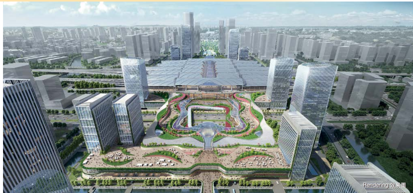
The sites adjacent to the Guangzhou South Railway Station, which will be developed into Guangzhou South Railway Station New Town, comprising office towers, a shopping mall, a hotel, residential units, serviced apartments and public transport facilities 廣州南站地皮將發展為「廣州南站新城」，匯聚寫字樓、商場、酒店、住宅、服務式公寓及公共交通設施等
