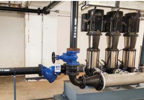
Shanghai IFC has a rainwater recycling system, which uses collected rainwater for irrigation 上海國金中心設有雨水回收系統，把收集所得雨水用作灌溉
