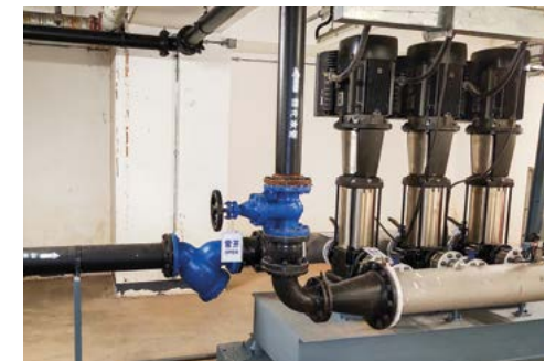
Shanghai IFC has a rainwater recycling system, which uses collected rainwater for irrigation 上海国金中心设有雨水回收系统·把收集所得雨水用作灌溉
