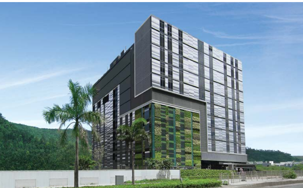
MEGA Plus in Tseung Kwan O started operating in 2017 and is located near SUNeVision's upcoming new data centre site, TKOTL 131. They will create significant synergy in operations and infrastructure investment 位於將軍澳的MEGA Plus於2017年開始運作·毗鄰新意網另一數據中心新用地(TKOTL 131)·兩者將於營運和基建投資方面產生重大的協同效應
