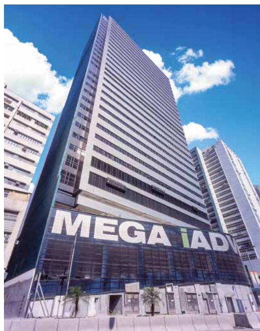
MEGA-i's revitalization project will substantially boost SUNeVision's connectivity business growth MEGA-i的优化工程将大幅提升新意网的网络连接业务发展
