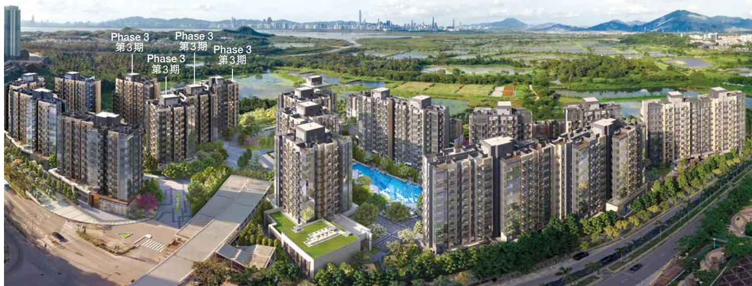
The above image was taken from some height above the Phase of the Development on 20 June 2019 and has been processed with computerized imaging techniques. The general appearance of the Phase of the Development has been merged and added by computer rendering techniques and processed with computerized imaging techniques, in order to illustrate the general appearance of the environment, structures and facilities surrounding the Phase of the Development. The image does not illustrate the final appearance or view of or from the Phase of the Development or any part thereof and is for reference only. The Phase of the Development was still under construction when the image was taken. The approved building plans of the phases of the Development might be revised from time to time and the details of the Phase upon completion may be different from the information contained in this image and are subject to the plans finally approved by the relevant Government departments. There will be other completed and/or uncompleted buildings and facilities surrounding the Phase of the Development and the district and surrounding environment, building and facilities might change from time to time. The Vendor does not give any offer, undertaking, representation or warranty whatsoever, whether express or implied as to the environment, structures and facilities in the district or surrounding the Phase of the Development. The fittings, finishes, appliances, decorations, plant, landscaping and other objects in the image may not appear in or the view may not be seen in or from the Phase of the Development or its surrounding area. They are for reference purpose only and do not constitute any offer, undertaking, representation or warranty whatsoever, whether express or implied, on the part of the Vendor regarding the Phase or the Development, their surrounding environment, structures and facilities. The Vendor also advises prospective purchasers to conduct on-site visit(s) for a better understanding of the development site, its surrounding environment and the public facilities nearby.
