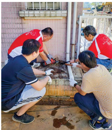
The SHKP Volunteer Team removes roots extending to the raised platform and near the drains in Green Garden to prevent clogged drains and cracks in the raised platform
