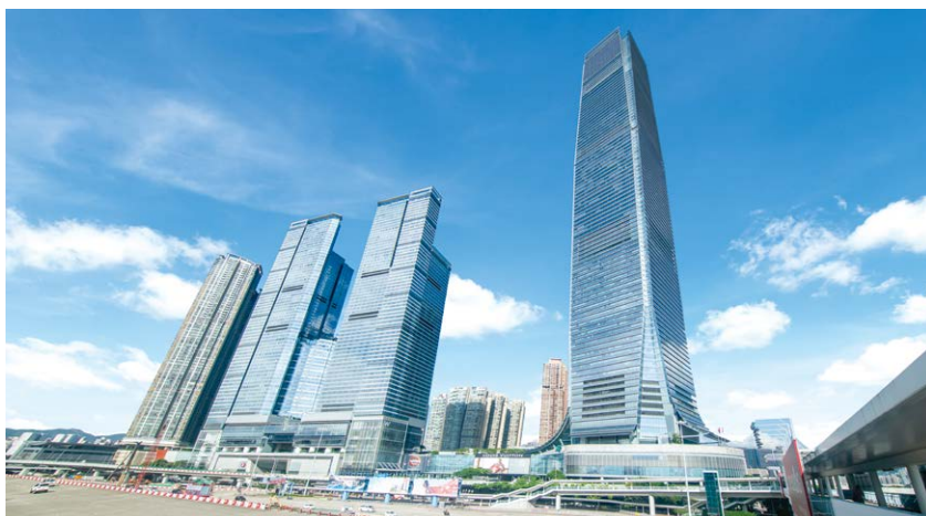
ICC receives the Hanson I&T Outstanding Award for its Smart Optimal Control of Central Cooling and Air Conditioning System project 環球貿易廣場憑著「智慧優化空調控制系統」項目奪得「卓越創科擘神獎」
