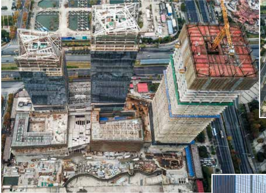
The first phase of the project will be completed by the end of 2018 (site photos taken on 30 November 2017)
