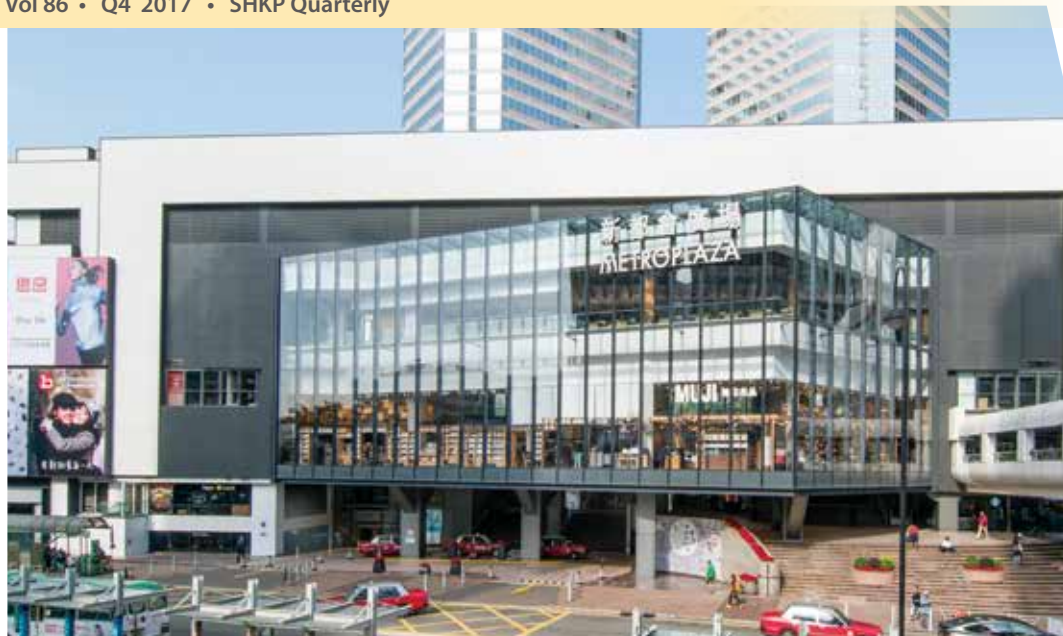
The glass facades give Metroplaza a brand new facelift 新都会广场外墙以全落地玻璃幕墙设计·感觉焕然一新
