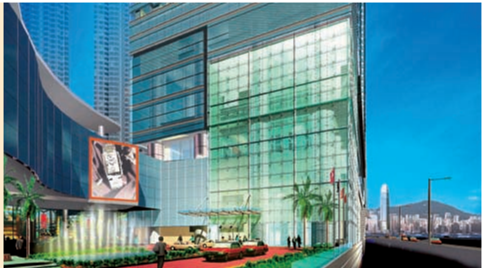
Works on the residential units and serviced apartments in the first phase of the Kowloon Station Development are underway.
