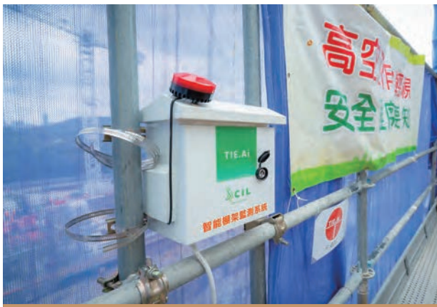
○ Hong Kong's first smart scaffolding monitoring system TIE.AI, developed by Sanfield
