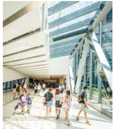
YOHO MALL is the convergence of three retail podiums linked by footbridges, with direct connection to West Rail Yuen Long Station. 整个YOHO MALL以大型天桥连接三个基座商场，也可接驳至西铁元朗站，出入方便。
