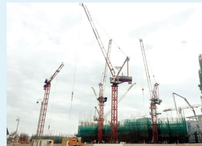
• The tower crane anti-collision system has been widely adopted at our construction sites to enhance safety
