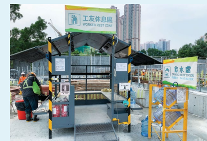
• Mobile resting station - a resting and gathering place for our construction workers
